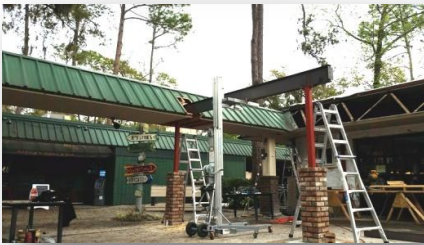
Custom Welding Design
